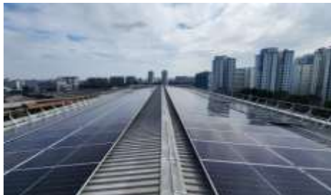
Solar panel installation at Kallang Basin 2 Cluster
